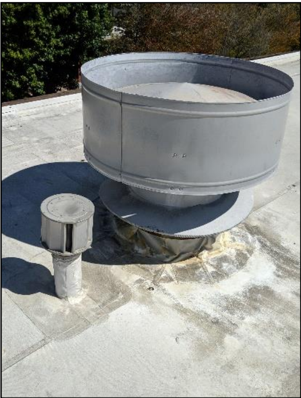
Mechanical Figure 12: Boiler Flue and Intake
