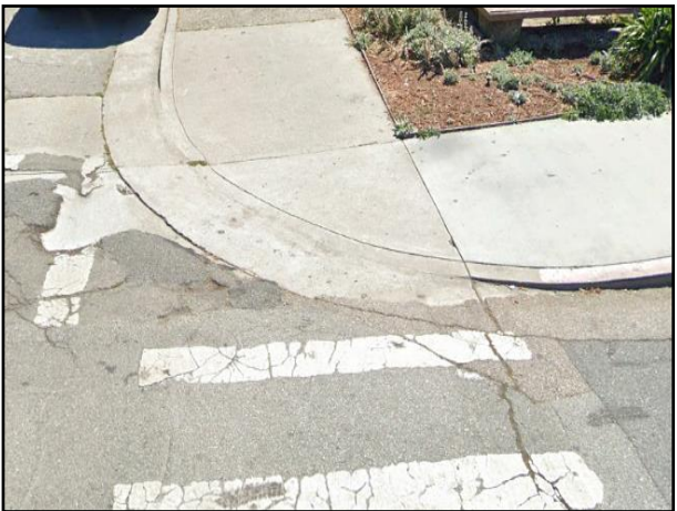
Civil Figure 6: Curb ramp on Locust & Center Street
