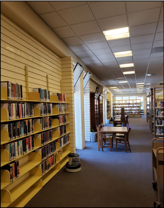
Concrete block walls at 1-story section
