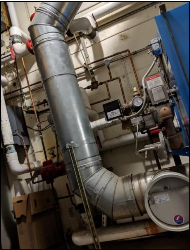
Mechanical Figure 5: Boiler Exhaust Flue
