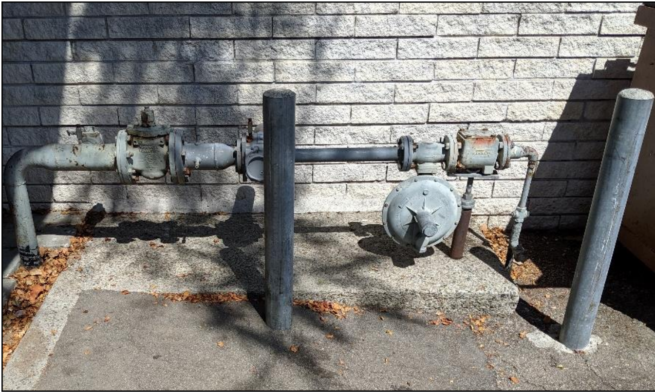
Mechanical Figure 13: Building Gas Meter
