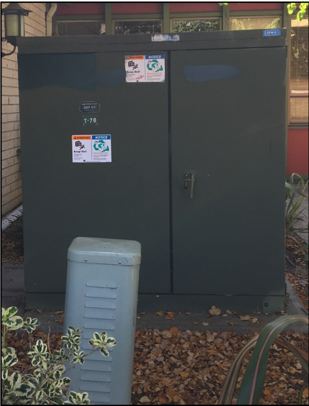
Electrical Figure 1: Utility Transformer
