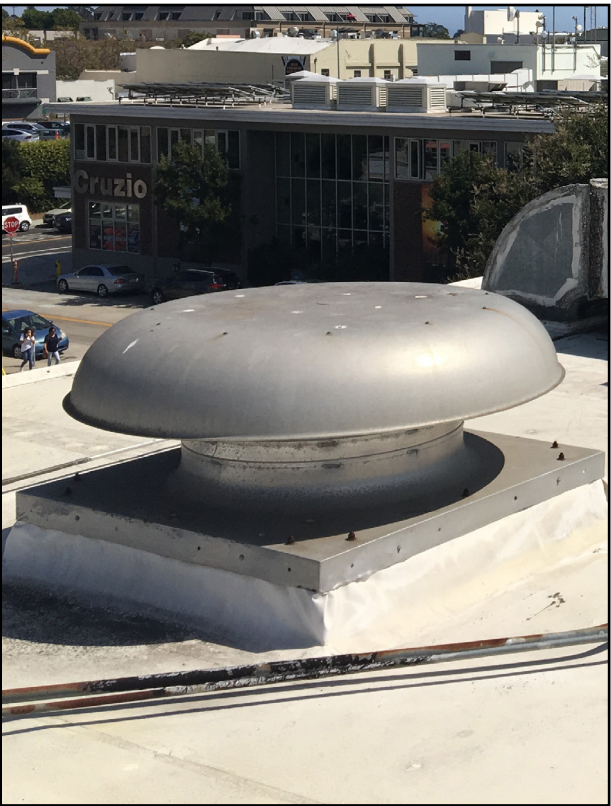
Mechanical Figure 9: Building Relief Hood
