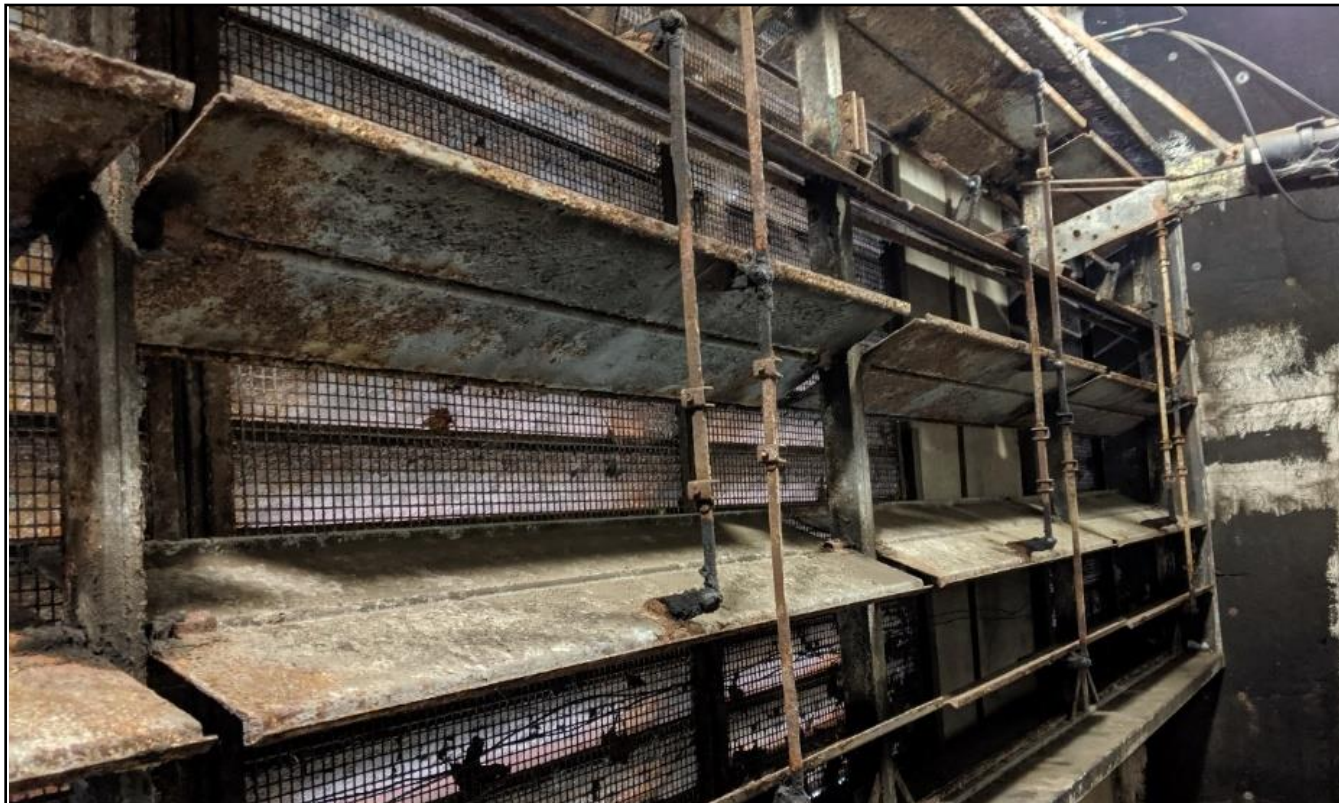
Mechanical Figure 1: AHU Modulating Mixing Dampers
