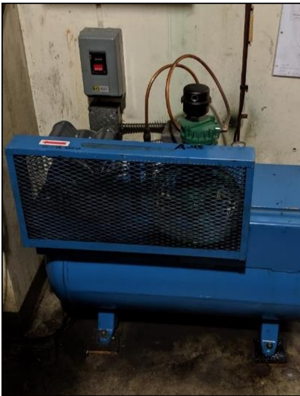
Mechanical Figure 14: Pneumatic Controls Air Compressor
