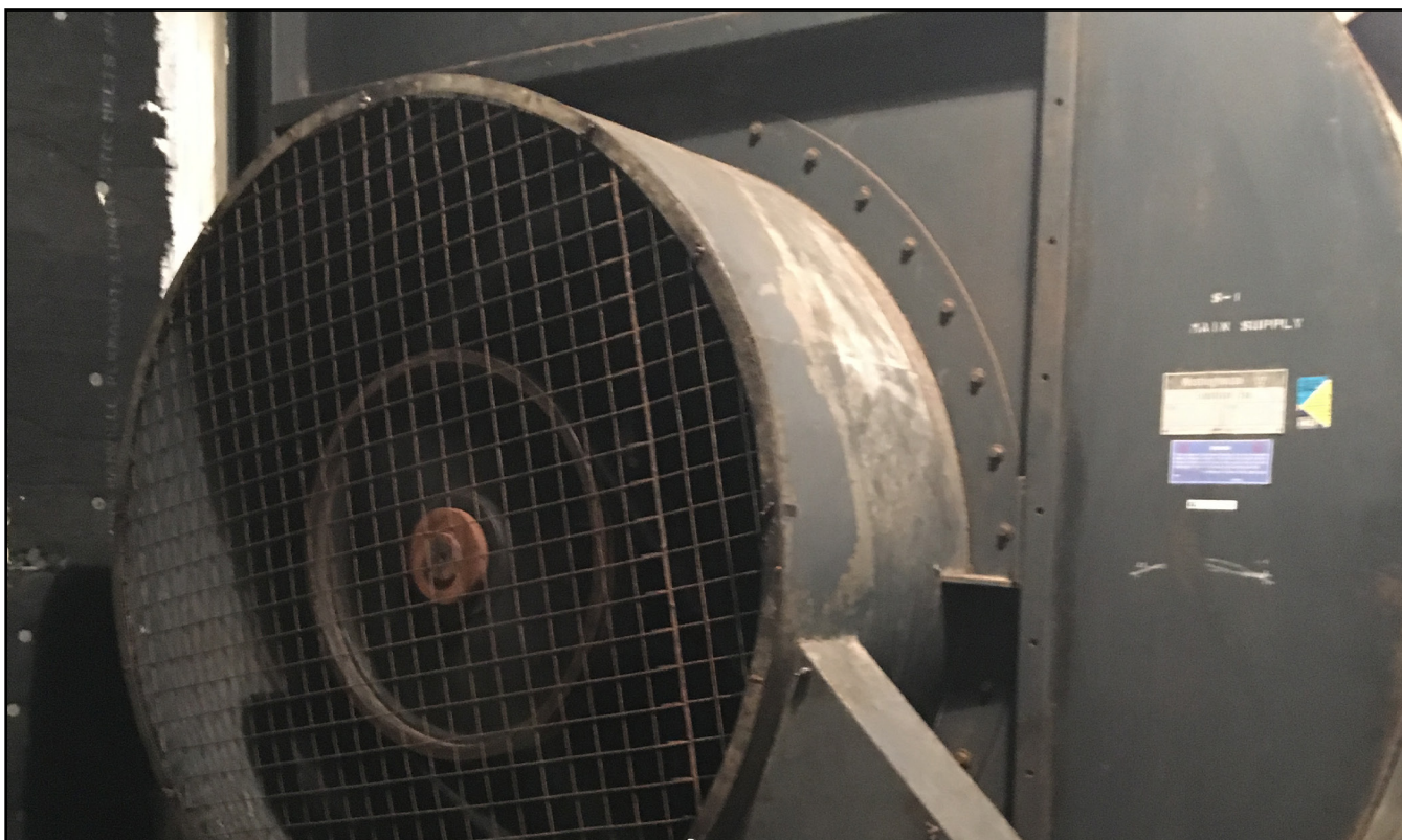
Mechanical Figure 2: AHU Plenum Supply Fan
