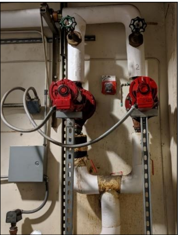
Mechanical Figure 4: Heating Hot Water Secondary Loop Pumps
