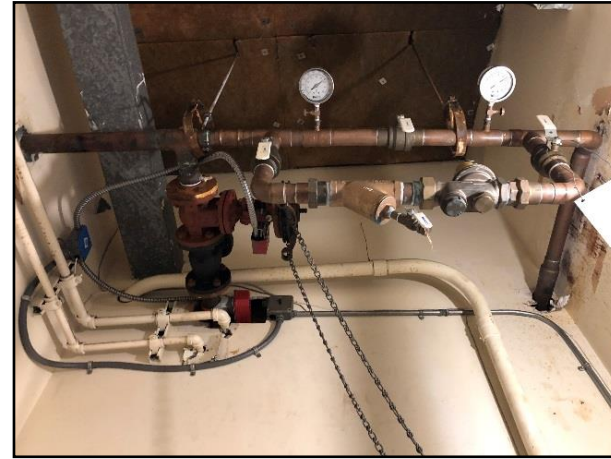
Civil Figure 8: Backflow preventer inside the building
