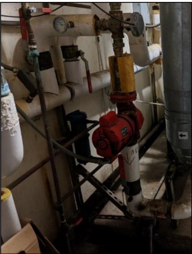
Mechanical Figure 6: Heating Hot Water Primary Loop Pump
