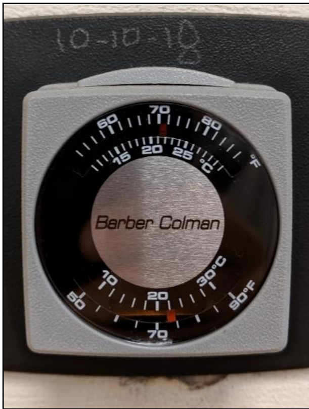
Mechanical Figure 15: Pneumatic Thermostat
