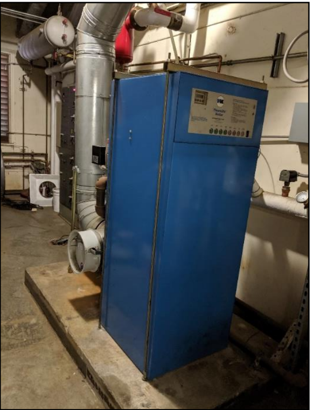
Mechanical Figure 3: Gas Fired Heating Hot Water Boiler
