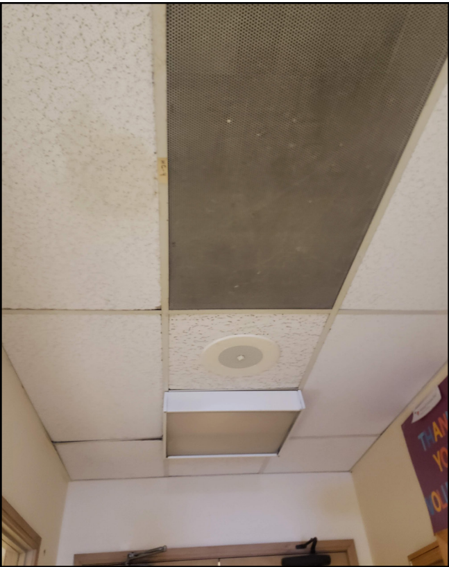
Deteriorating and water damaged ceilings
