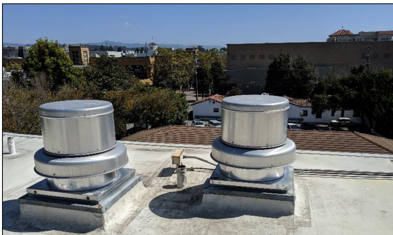
Mechanical Figure 8: Building General Exhaust Fans
