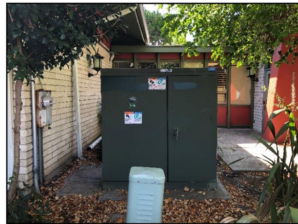
Civil Figure 10: PG&E transformer on Locust Street
